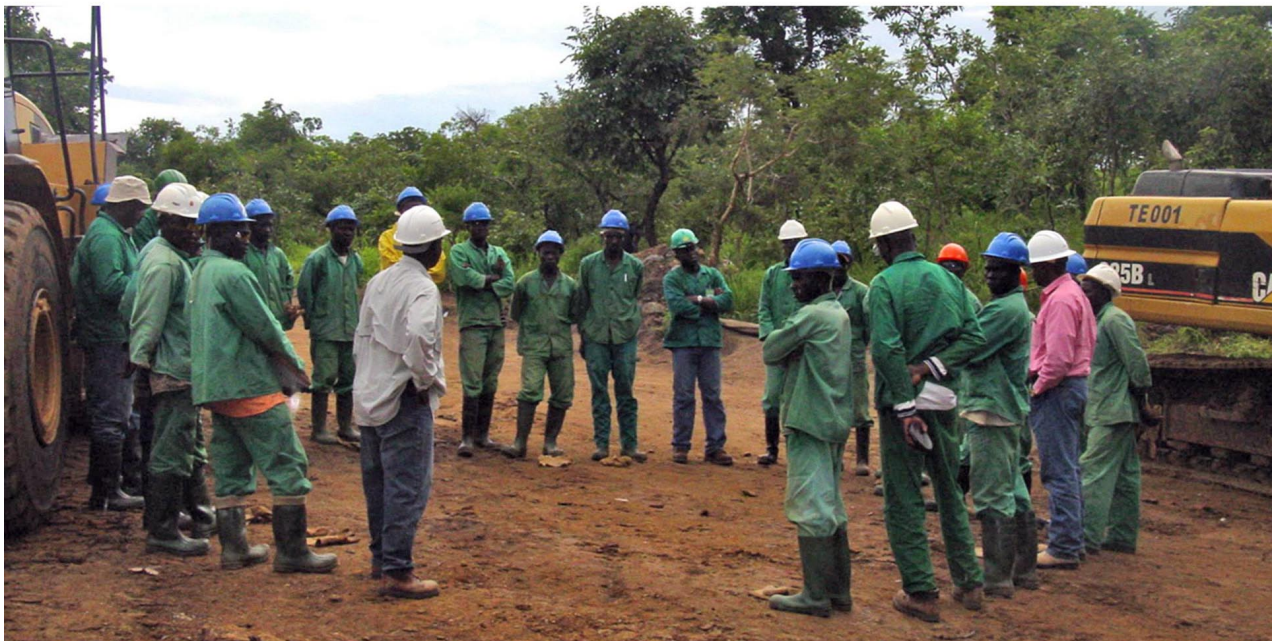
In Cameroon, the Project has been conducting pipeline right of way maintenance operations by hiring local contractors to do the work. Bantou Expertises Conseils, shown here, is one of several such contractors. Proprietor Guillaume Nde says he has hired over five dozen residents from nearby villages.
